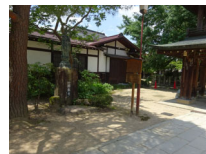
005_① 鐘樓門・遠景005
