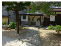
003_① 鐘樓門・遠景003
