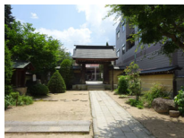
001_① 鐘樓門・遠景001
