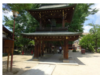
006_① 鐘樓門・遠景006
