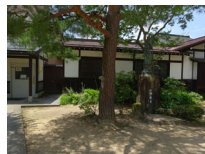
004_① 鐘樓門・遠景004
